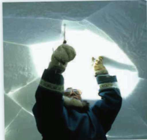
The window in this igloo is made of sea ice.
